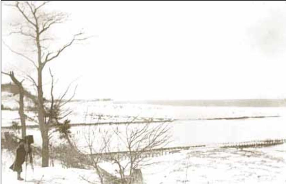
A project to build a harbor of refuge at Portage Lake, of which the Channel would be a part, was adopted in 1879 by the United States Government. Work began on the wooden substructures of the outer piers in 1883 and continued through 1901. The cement superstructures were added to the outer piers in 1939-1940; the
