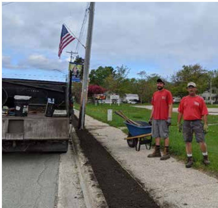
Soil preparation done by Larsen's Landscaping (weed control, soil amendment).
